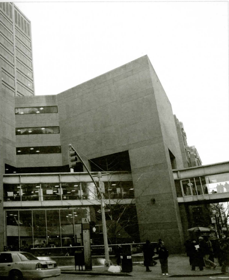
Avenue. Another bridge crosses 68th Street to the North Building and Thomas Hunter Hall.
