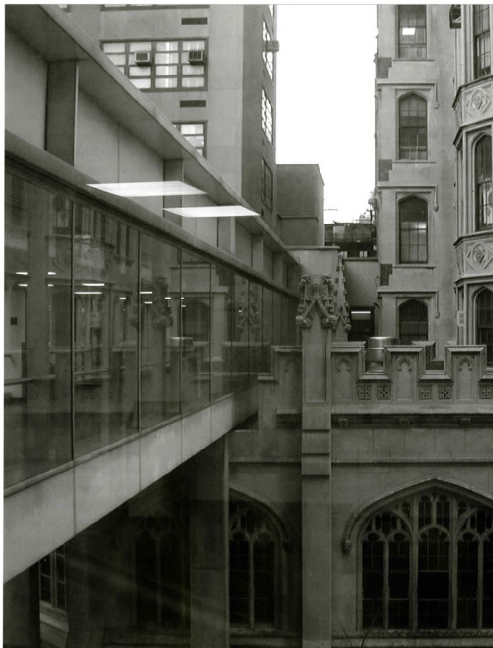
Skybridge from the West Building to the North Building and Thomas Hunter Hall
